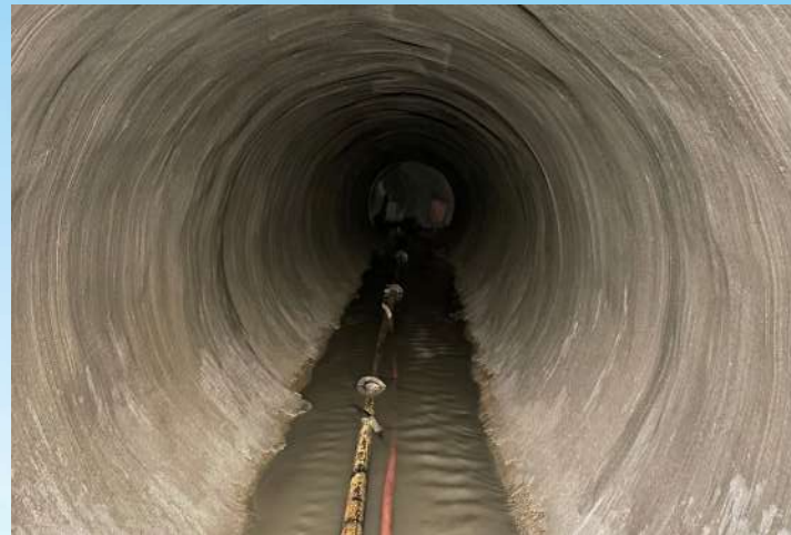
Spin Cast Geopolymer Lining
