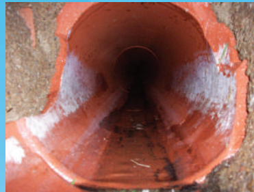
Before CIPP rehabilitation
